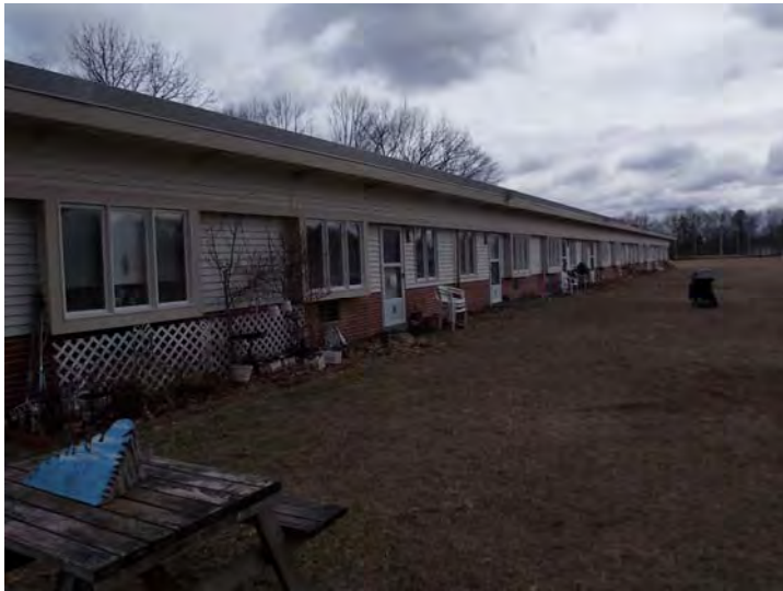
Vinyl siding is also used to clad portions of the exterior walls.
