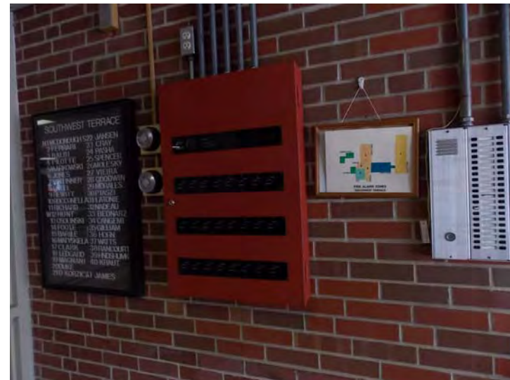
This is the fire alarm control panel (FACP).
