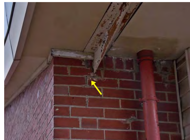
A close-up of a step crack along a section of a brick exterior wall.
