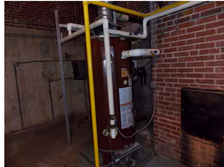
This is the DHW tank that serves the common areas. Each apartment has its own DHW tank.
