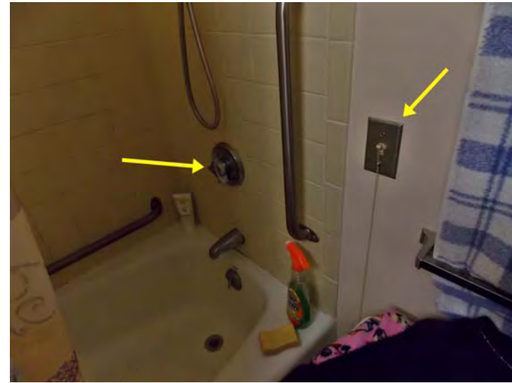
Bathrooms also include an anti-scald mixing valve (over the tub), and a medical emergency pull cord (on right).
