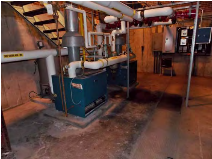
This pair of gas-fired boilers produces hydronic heat for the facility.
